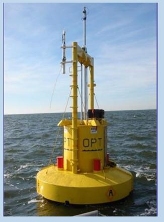
**Wave Power** is created by the wind out to sea blowing over the surface of the water, creating a swell due to friction. Rotation of water particles within the swell causes the wave to move forward. Wave energy involves converting the motion of the wave into electricity. It is more predictable than wind power. Wave power reduces as the water shallows, but with 50m+ depths within a couple of miles of the shore, Guernsey can take advantage of this resource.
